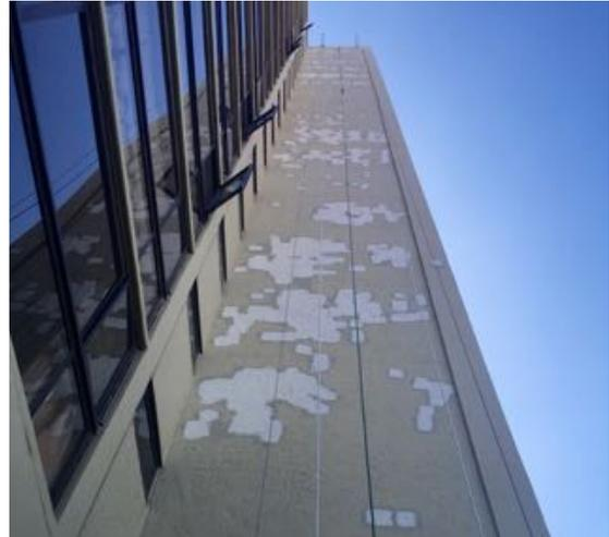
taken down to concrete and patched ( see picture ). Once the patches cured the entire wall was painted. Phase 2 - the rest of the residence tower - has been approved by the Board, with Raymond's scheduled to proceed upon Phase 1 completion.
